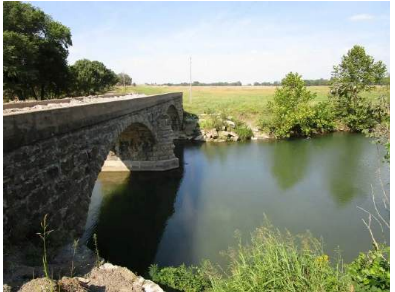
Stone Arch Bridge In Cowley County
